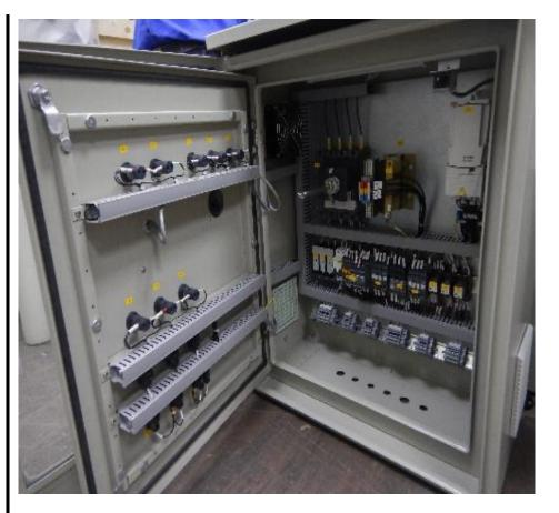
Starter - VFD with DOL Bypass Starter
